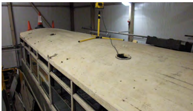
Above: The roof woodwork is in very good condition.
